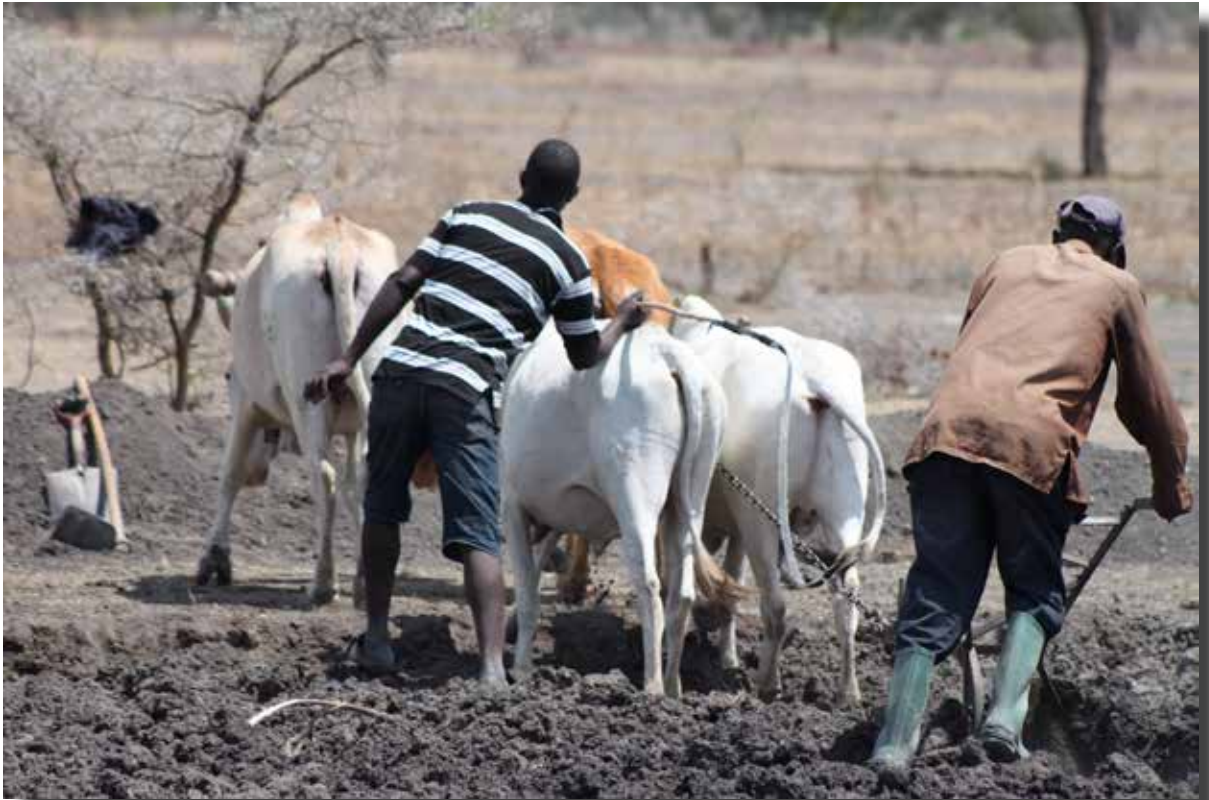
Figure 1: Ox-drawn plough is used to soften the soil in the excavation area of a dug-out pond
