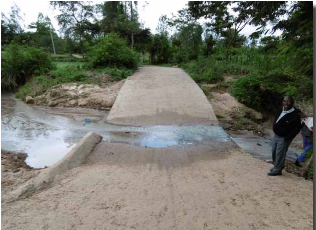
Figure 7: Small drift at narrow river section in Kitui, Kenya
