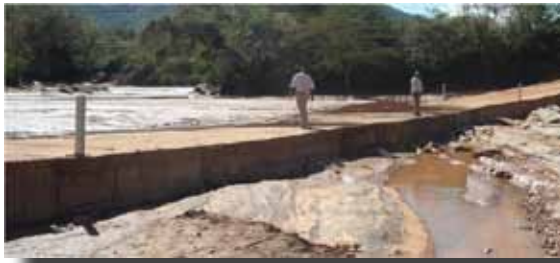
Figure 6: Non-vented drift crossing a river in Kenya
