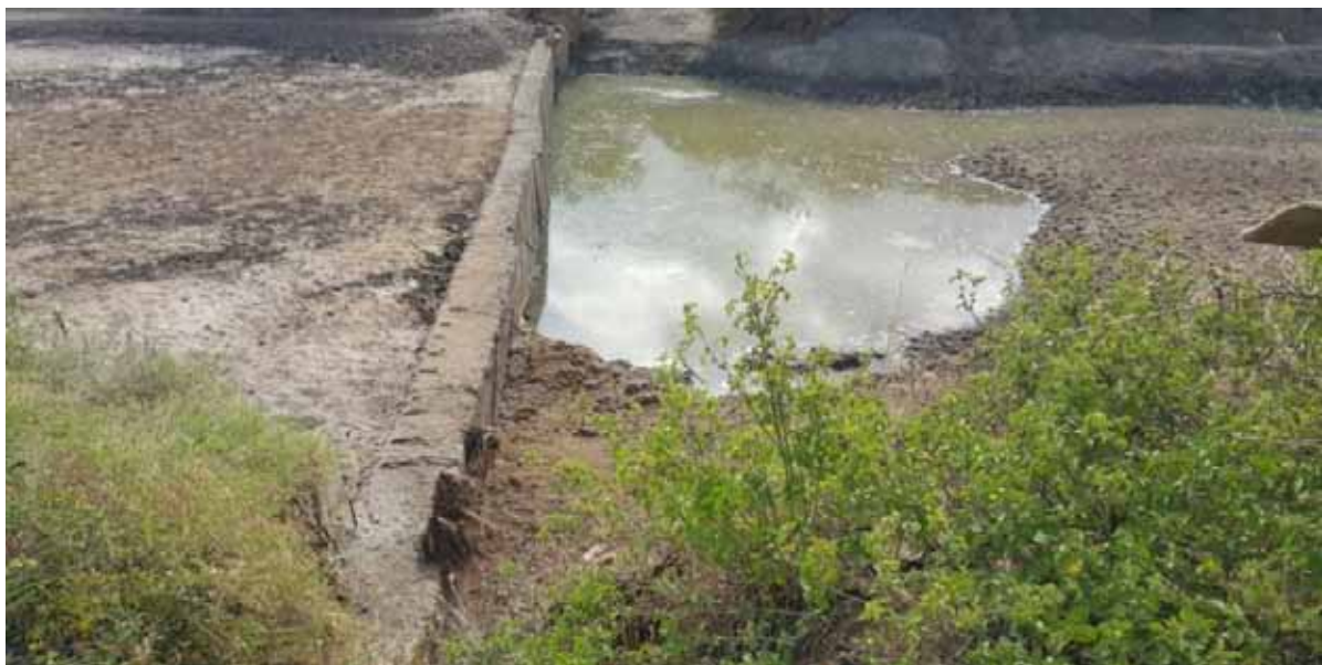
Figure 16: Example of a retaining wall, holding sand upstream
