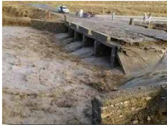
Figure 1: Example of vented bridge washed away by the force of the flood, Balochistan, Pakistan
