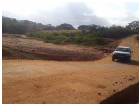
Figure 2: Example of non-vented drift, acting as sand dam to retain the sand upstream, Makueni, Kenya.
