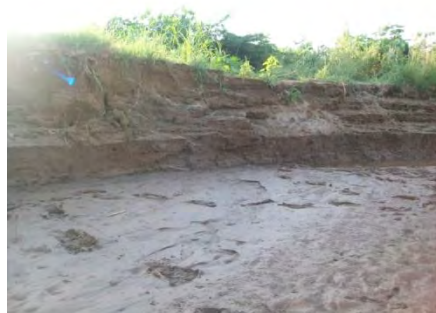
Fig (4): Erosion on the left bank of Old Geera gauging Station
