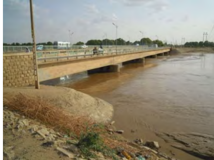
Fig (5): Right bank of Gash River at Kassala Bridge station
