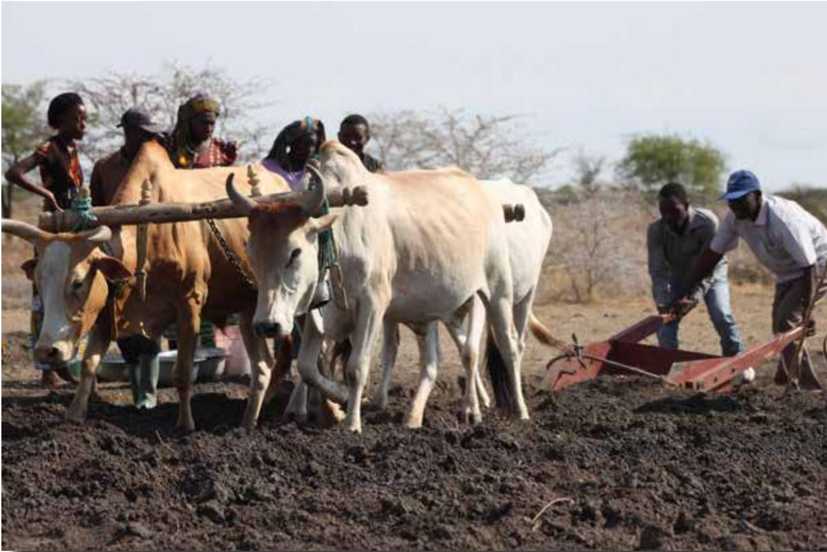
Figure 2: An ox-drawn scoop (locally constructed) is used to remove the soil from the excavation area and dispose it where the embankment will be established.
