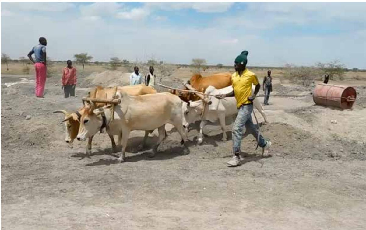
Figure 3: An ox-drawn compactor was built out of an old oil drum and is used to compact the embankments
